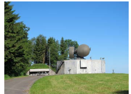
BL-64 'Hardened' T87 and adjacent Ops Bunker containing the LCP
